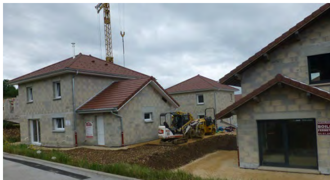
Construction neuve, Granges-Narboz
